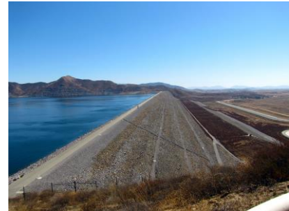
Figure 34: DVL West Dam
