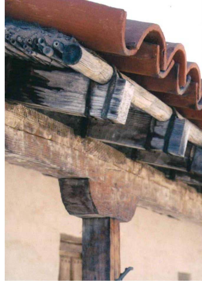
WOOD BEAM DETAIL W/ EXPOSED RFTERS
