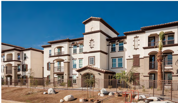
Figure 3.12 Heavier materials and textures shall be used lower on the building elevation to form the building base.
