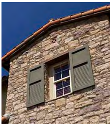
Figure 3.9 The minimum inset shall be 3 inches.
