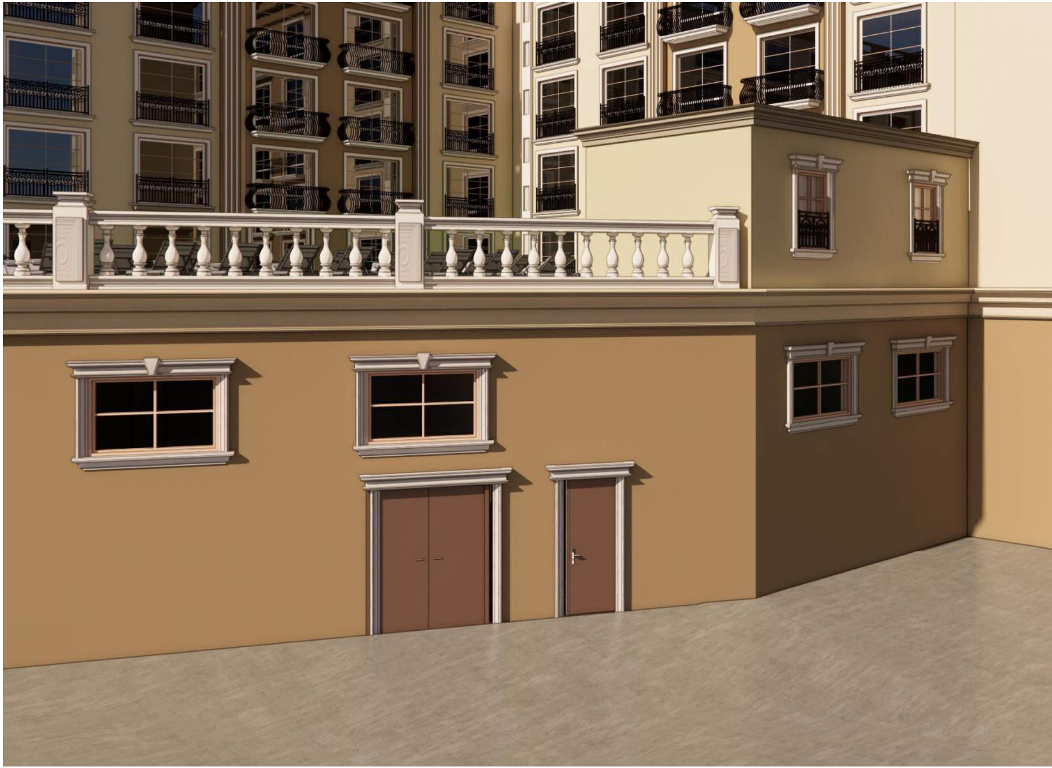
MECHANICAL & TRASH ROOMS
