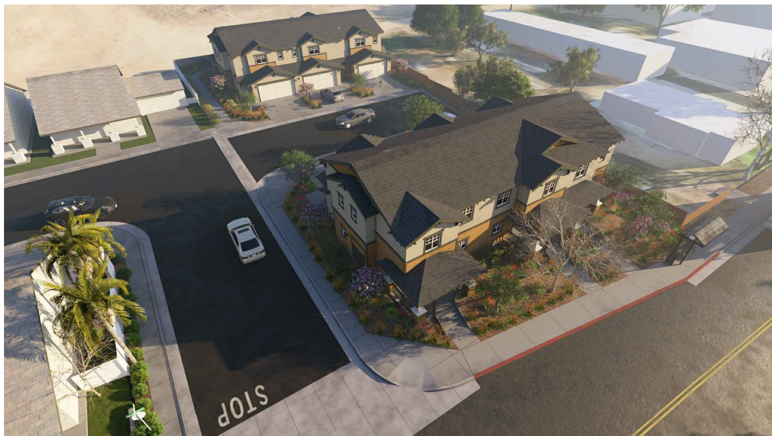
④ Front Left Aerial View
