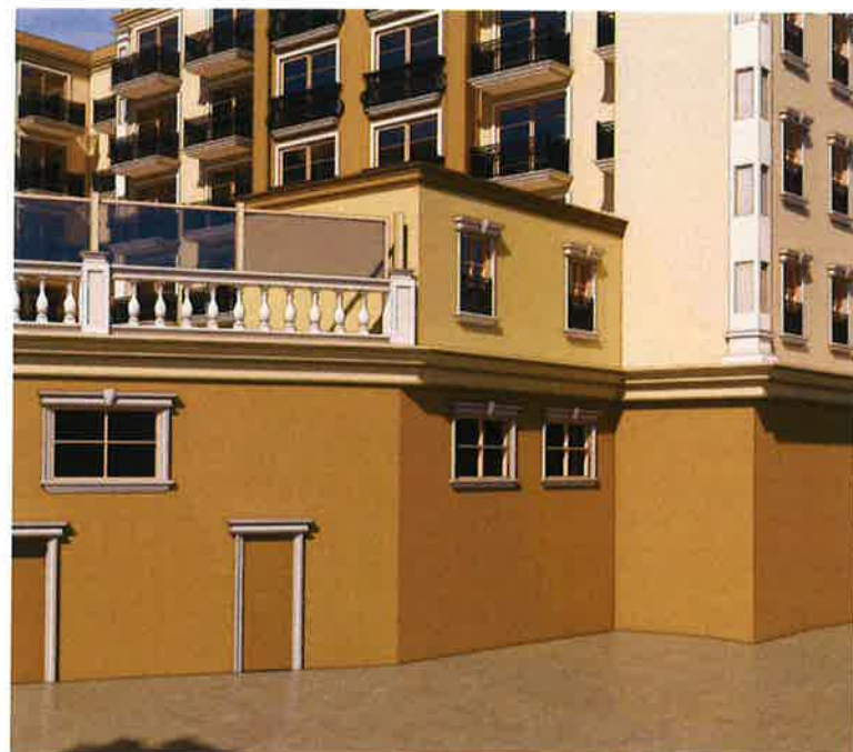
MECHANICAL & TRASH ROOMS
