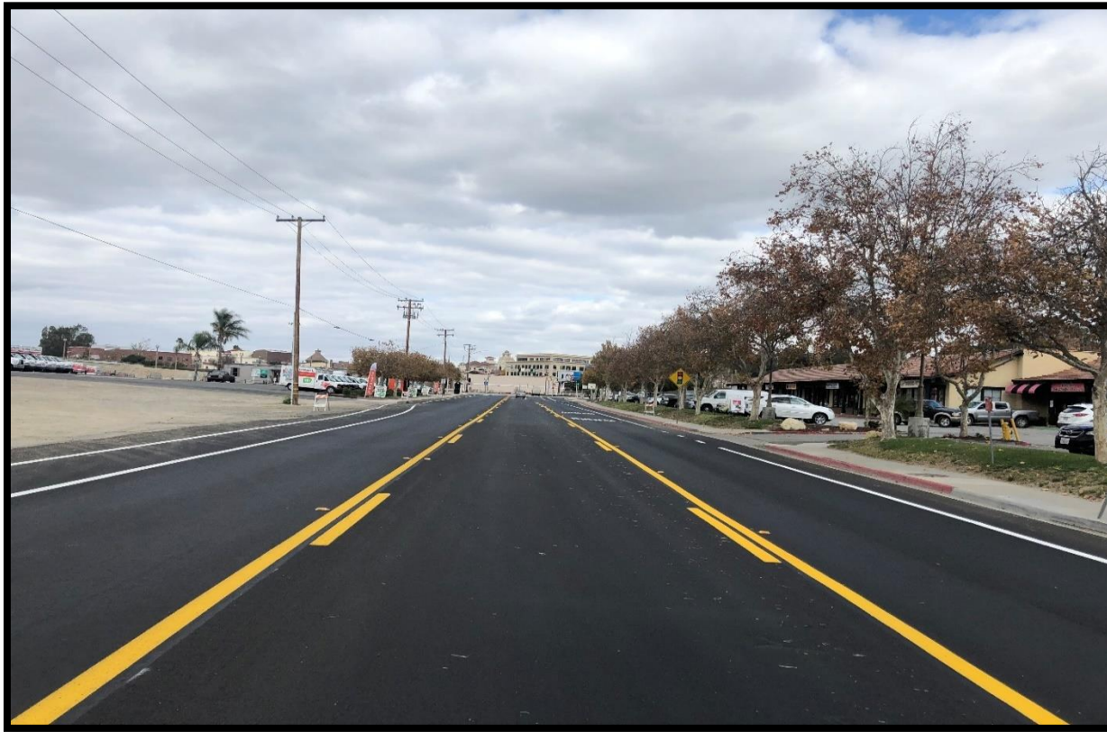
Road Resurfacing and Restriping – Old Town Front (First to Temecula Parkwa
